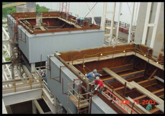
Widows Creek Scrubber Component Installation, June 2003
